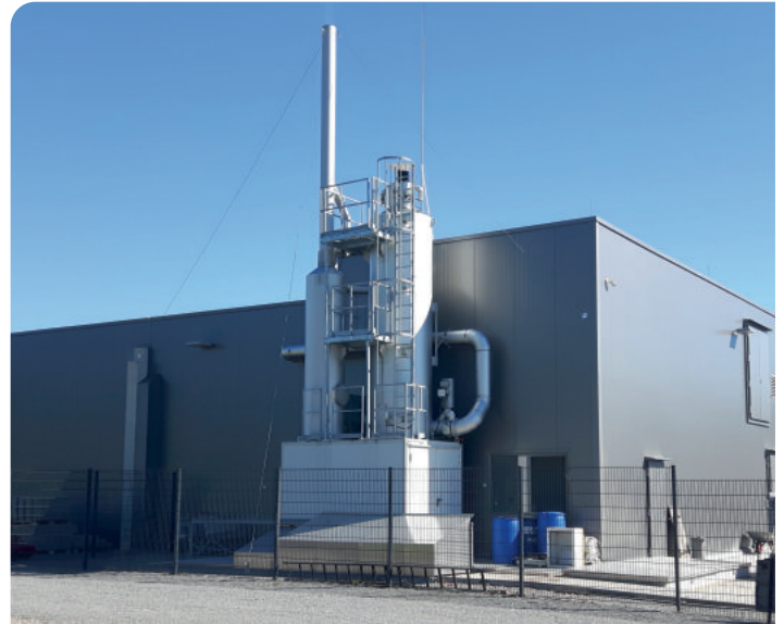
Fig. 3: The central air filter system has a smoke filter capacity of 3,000 m³/h and disposes the exhaust air of cold as well as hot smoke plants.
