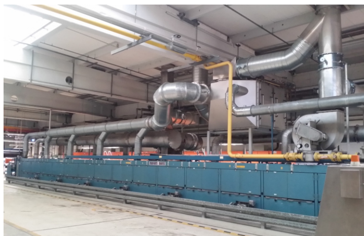
The integrated heat recovery technology can be designed to heat up the supply air of the stenter frame and process water.
