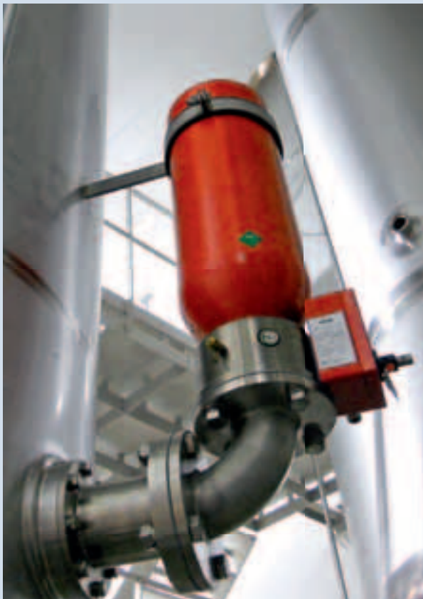
Additional safety through an explosion suppression system for explosive dust
