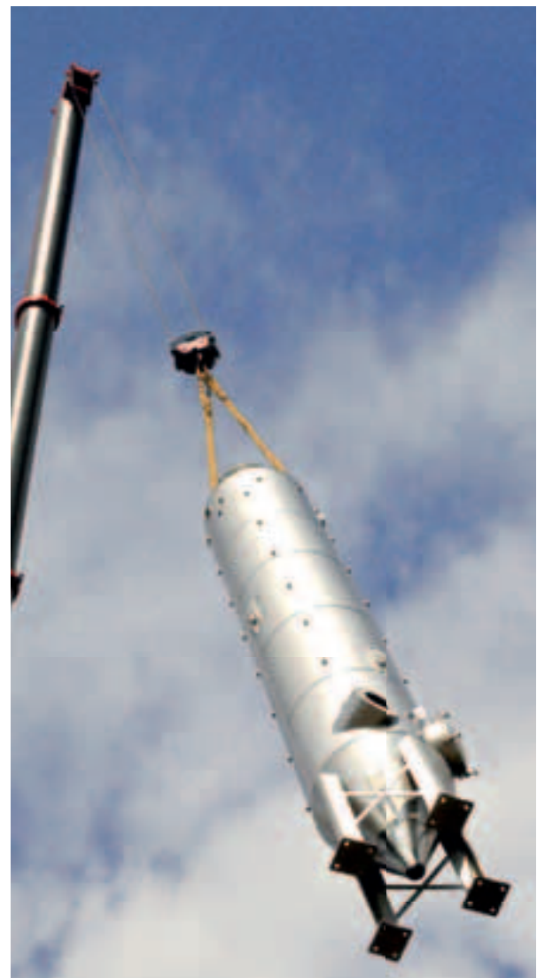
Insertion of a filter tube into a factory building
